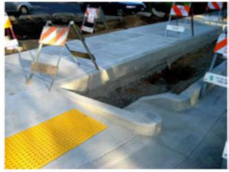
A bioswale is a landscaping element that collects rainfall as it runs off the pavement where the water can slowly soak into the ground, and water-loving plants help filter contaminants and improve water quality.
